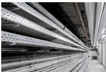
Cable trays, pipe installations
