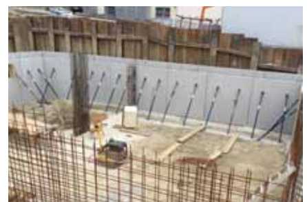
BTS M: Inclined supports / site facilities
